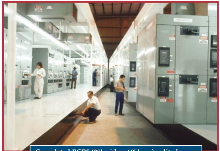
Completed PCR® (28' wide x 60' long) split along the length for shipment.
